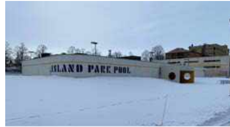
Island Park Pool East Entrance
