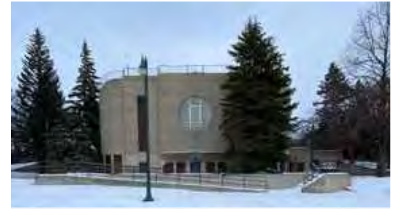
Historic Island Park Pool/Scherling Complex West Entrance
