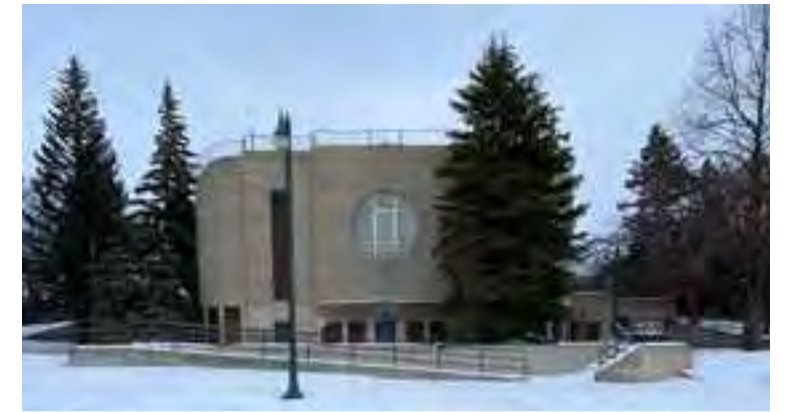
Historic Island Park Pool/Scherling Complex West Entrance
