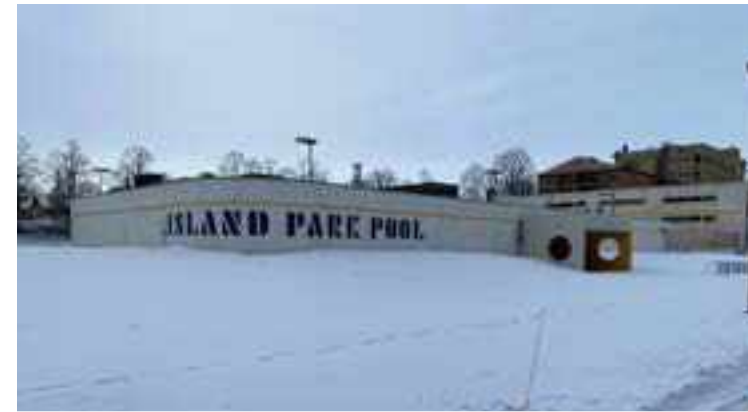
Island Park Pool East Entrance
